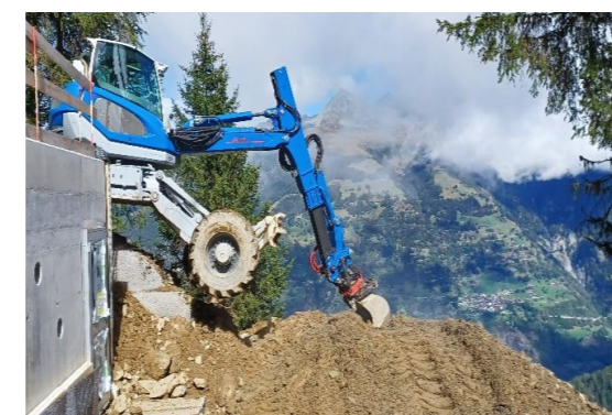
Remblayage – Station amont
