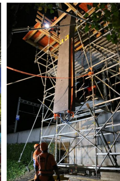
OCP – pose pilier BFUP
