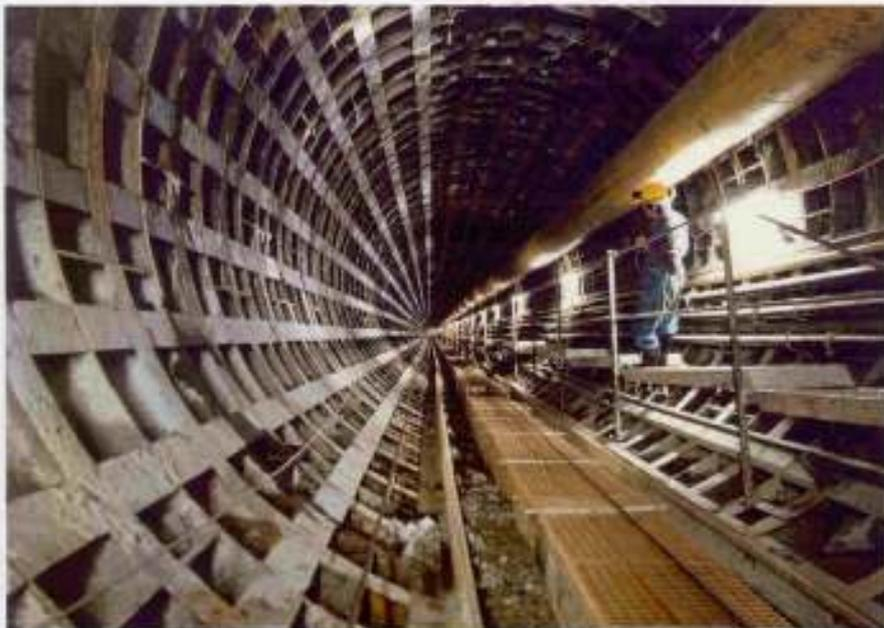
Lot D: Steel Segment Lining in inclined shaft F5 „Dzerjonna“
