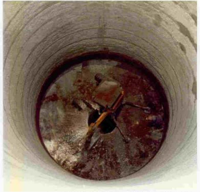
Surge Tank: Shaft sinking over 300m by drill and blast
