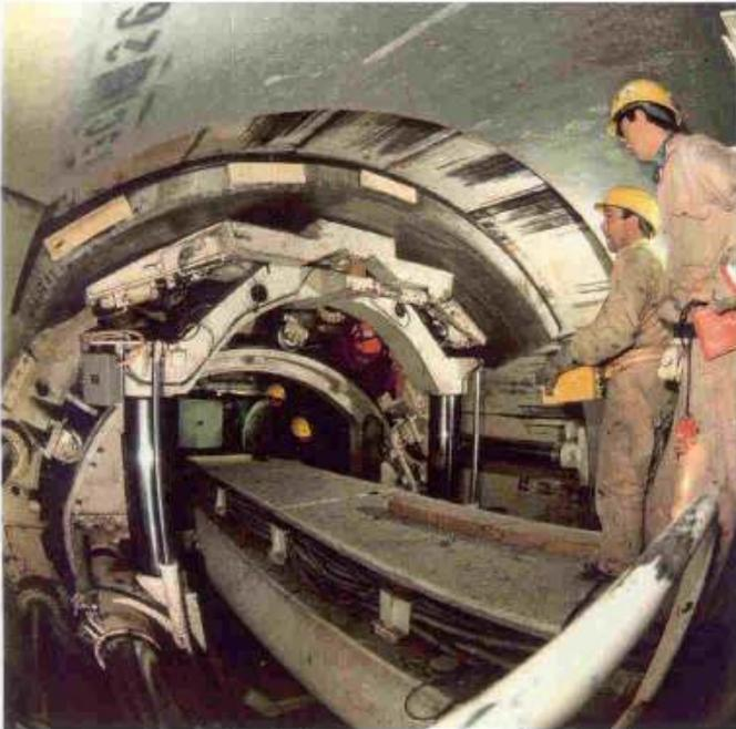
Lot C: Erection of concrete hexagonal segments
