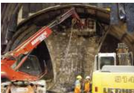
Excavation Station Bessières
