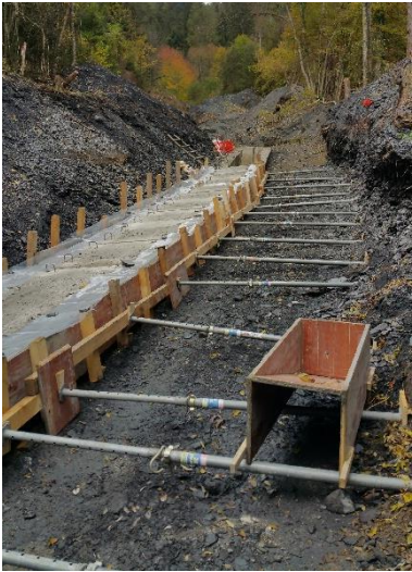
Coffrage bord dalle
